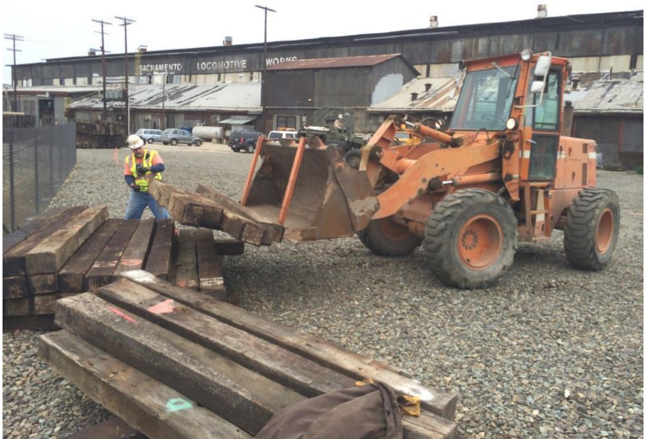
Mike F. stacking 10-foot ties by hand
