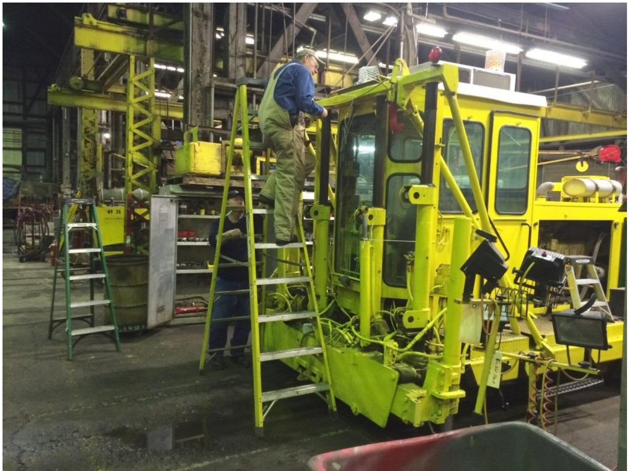
Gene and Cliff installing protective shields over the lights and horn on the new-old tamper
