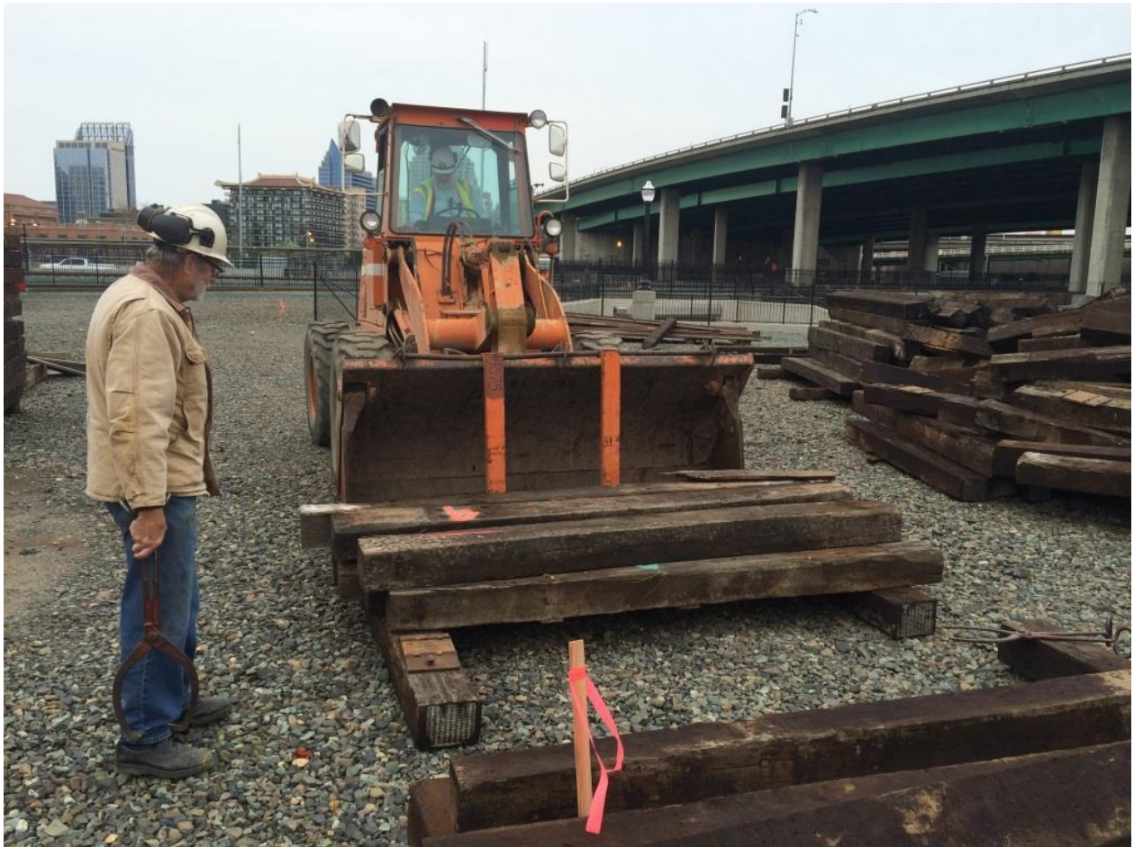
Alan, with tie-tongs in hand, works with Frank in the loader with the forks attachment moving loose ties
